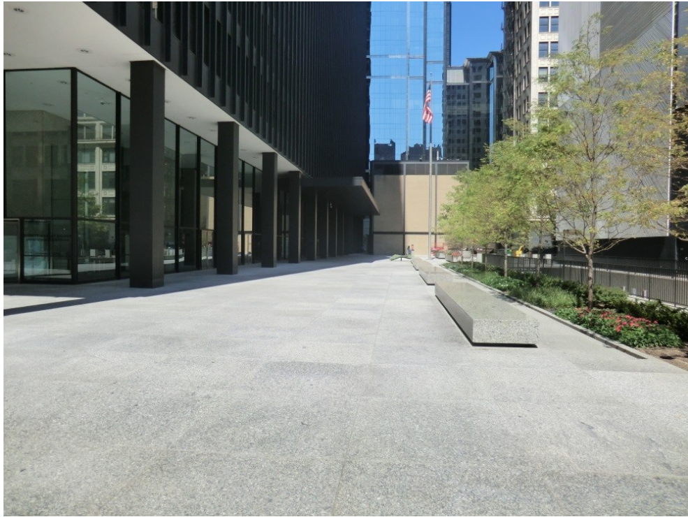
Figure 13: The plaza provides additional standoff distance for the buildings
