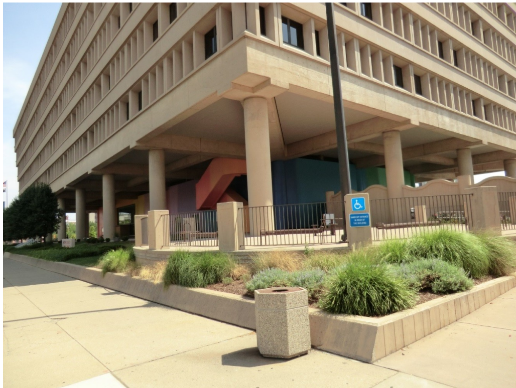
Figure 37: Minton-Capehart Federal Building-West view
