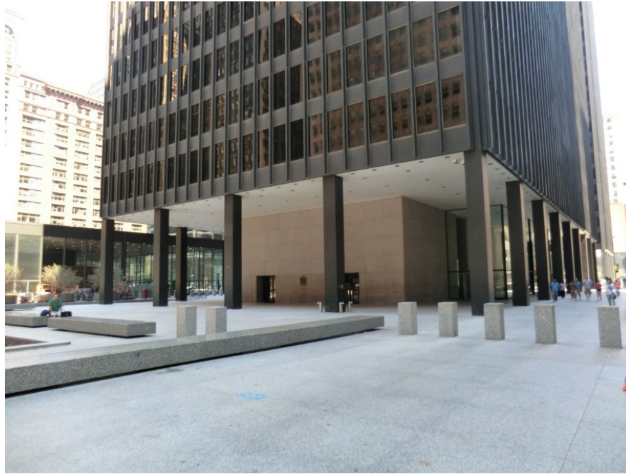
Figure 12: Public seating also serving as a barrier
